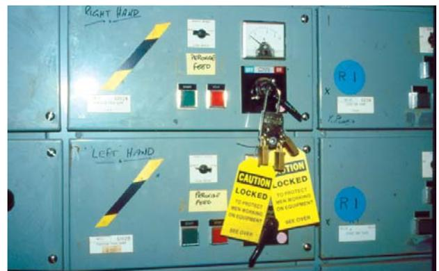
If locking-off facilities are not provided on the relevant switch then a locked DB door or locked switch-room door is acceptable provided the key or combination is unique, and is retained by the person doing the work.
