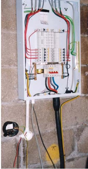
An electrician working on a new-build construction project installed the 3-phase and neutral distribution board shown in the photograph. He energized the supply to the distribution board before the circuits connected to it were complete, to provide a supply to a socket-outlet.
